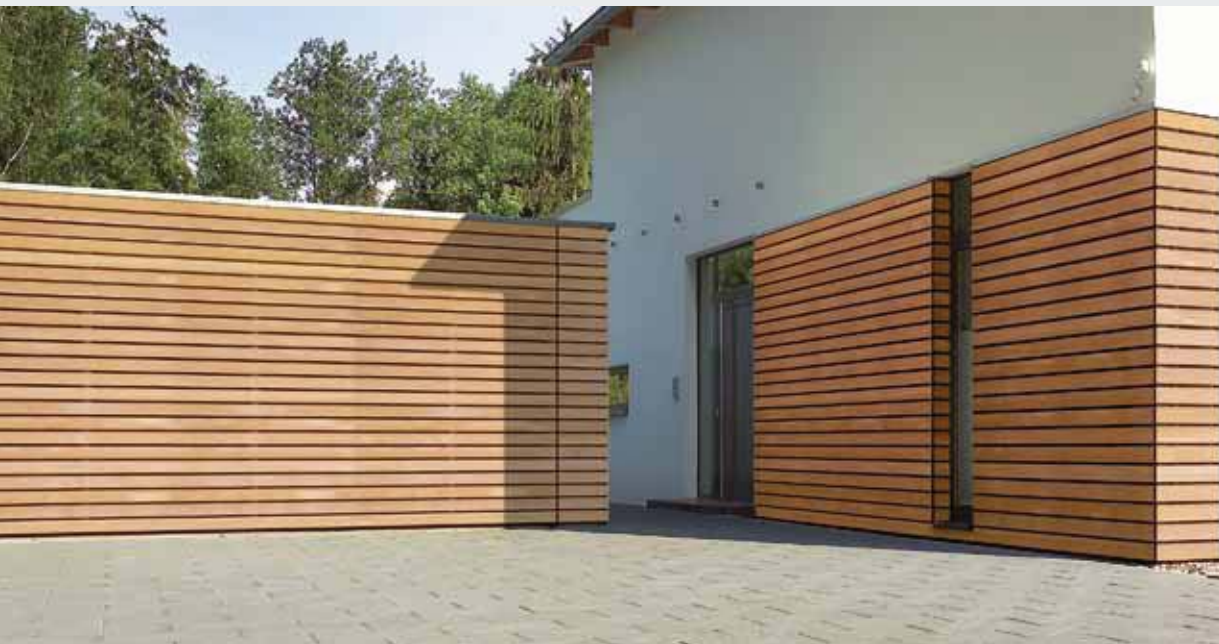
On-site cladding with timber panels
