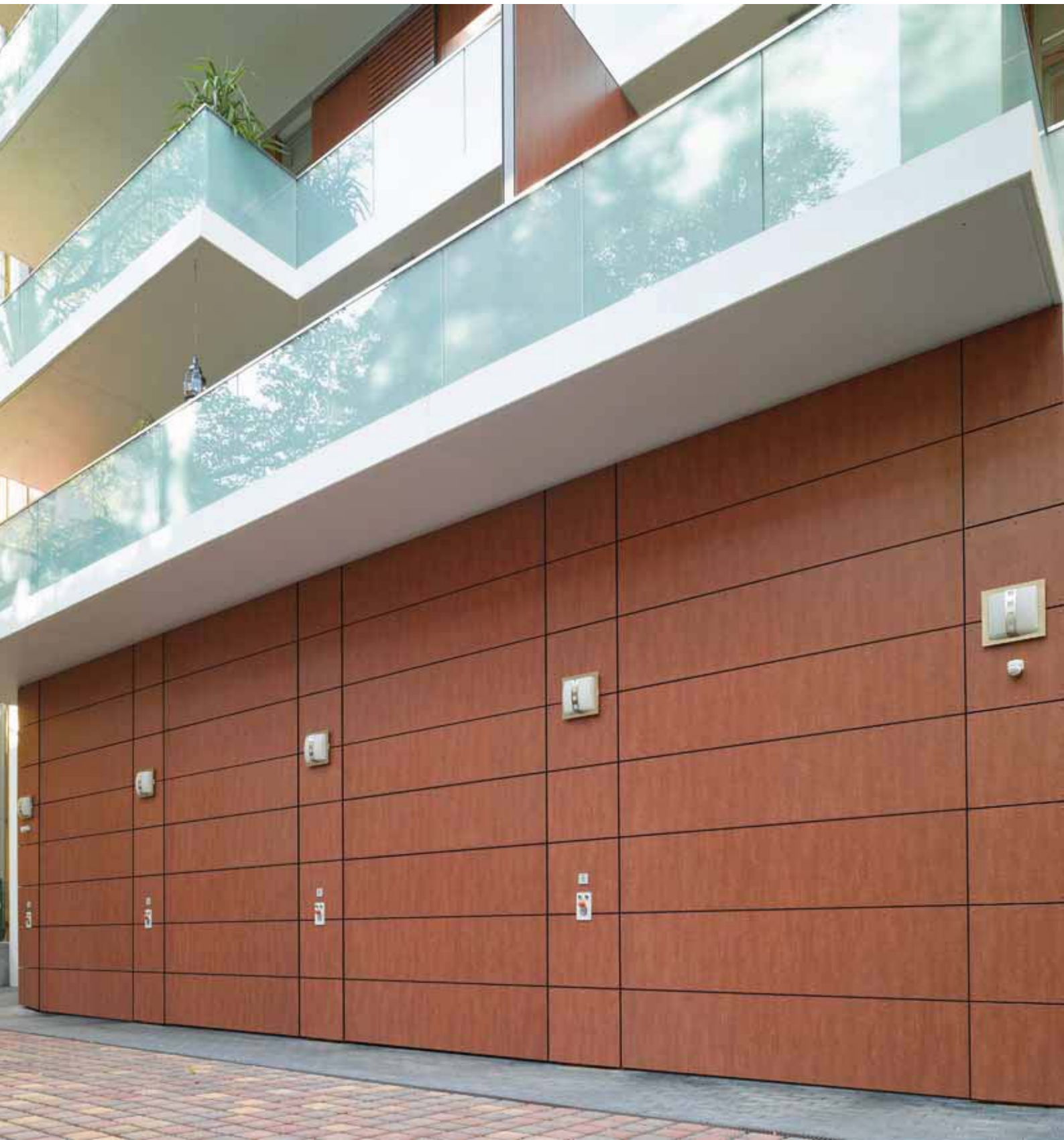
On-site cladding with laminated timber boards
