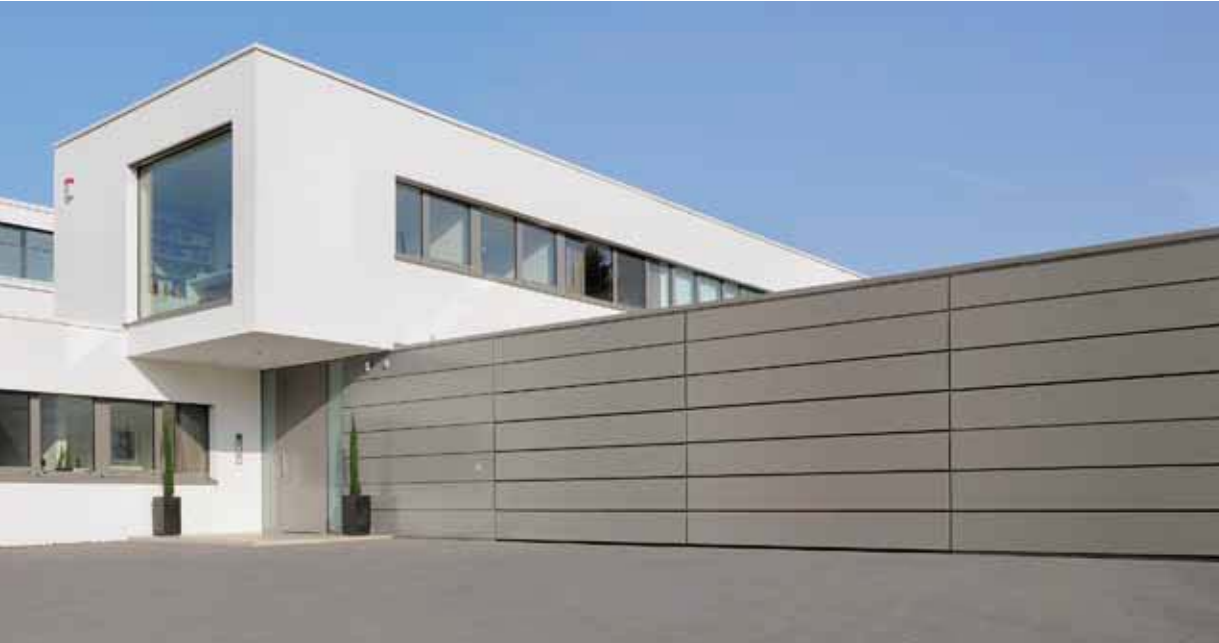
On-site cladding with aluminium compound board
